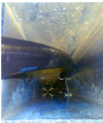
View of vibration dampner inside an aluminum light pole.
