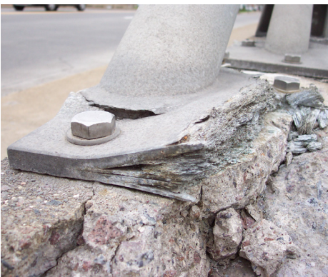
Corrosion at the base of a pole.
